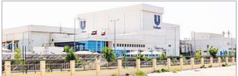
● The Unilever Dubai Personal Care factory produces 20 per cent of its energy between solar PV and solar thermal plants
